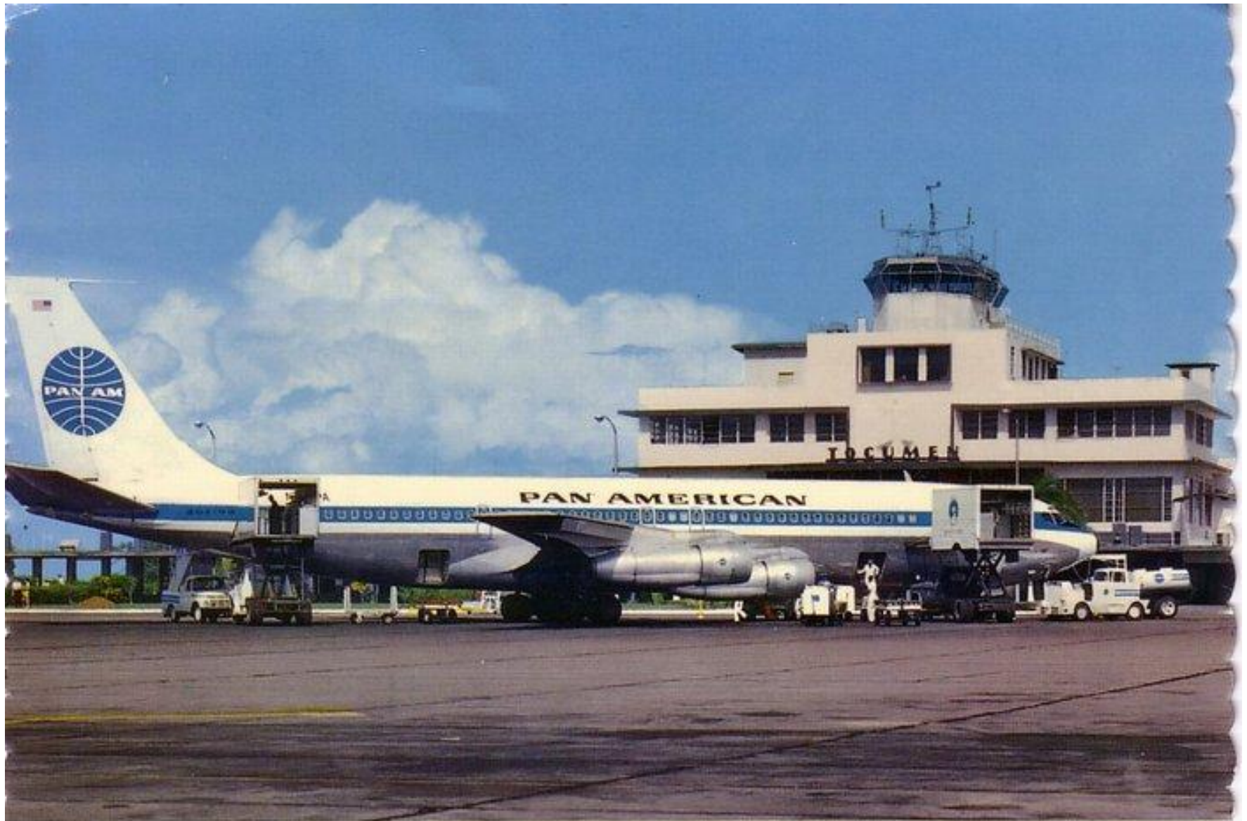
Tocumen International Airport
